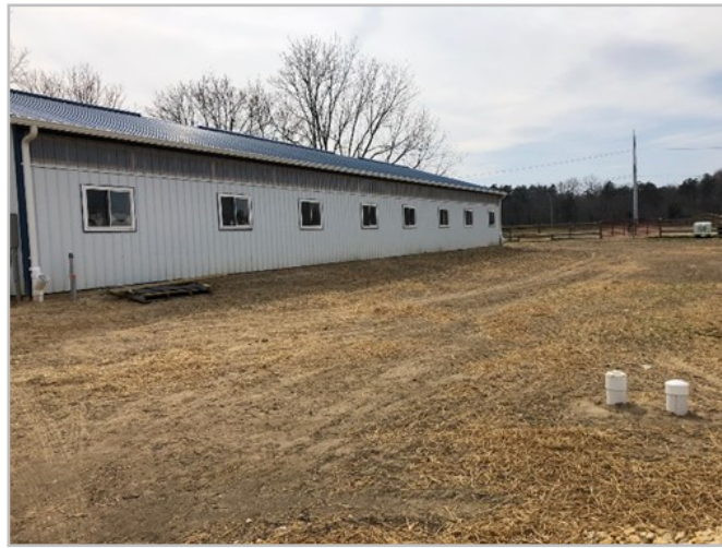
Roof runoff installed on a large horse stable with stormwater outletting into an underground cistern
