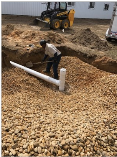
Roof runoff installed on a large horse stable with stormwater outletting into an underground cistern
