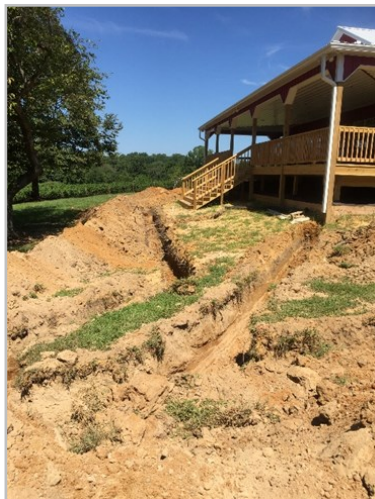
Roof runoff installed on a winery and tasting room with the water outletting into a stormwater management pond
