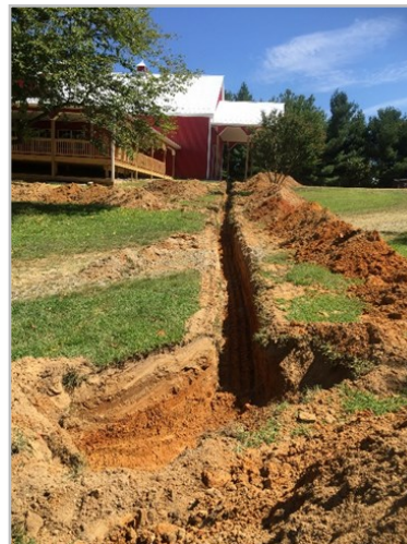
Roof runoff installed on a winery and tasting room with the water outletting into a stormwater management pond
