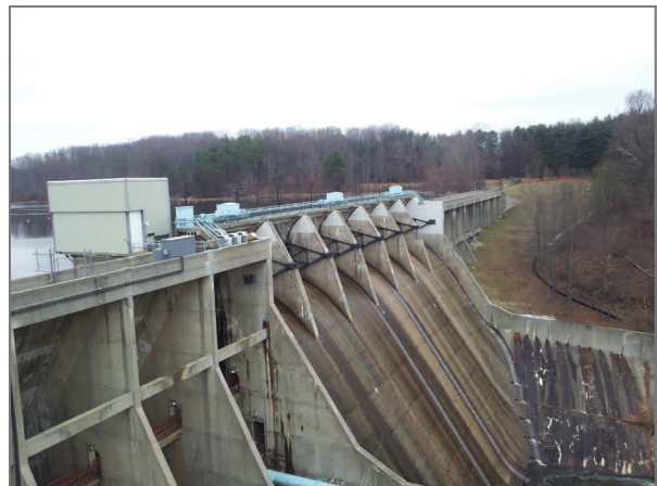
A view of the Duckett Dam concrete spillway system.
